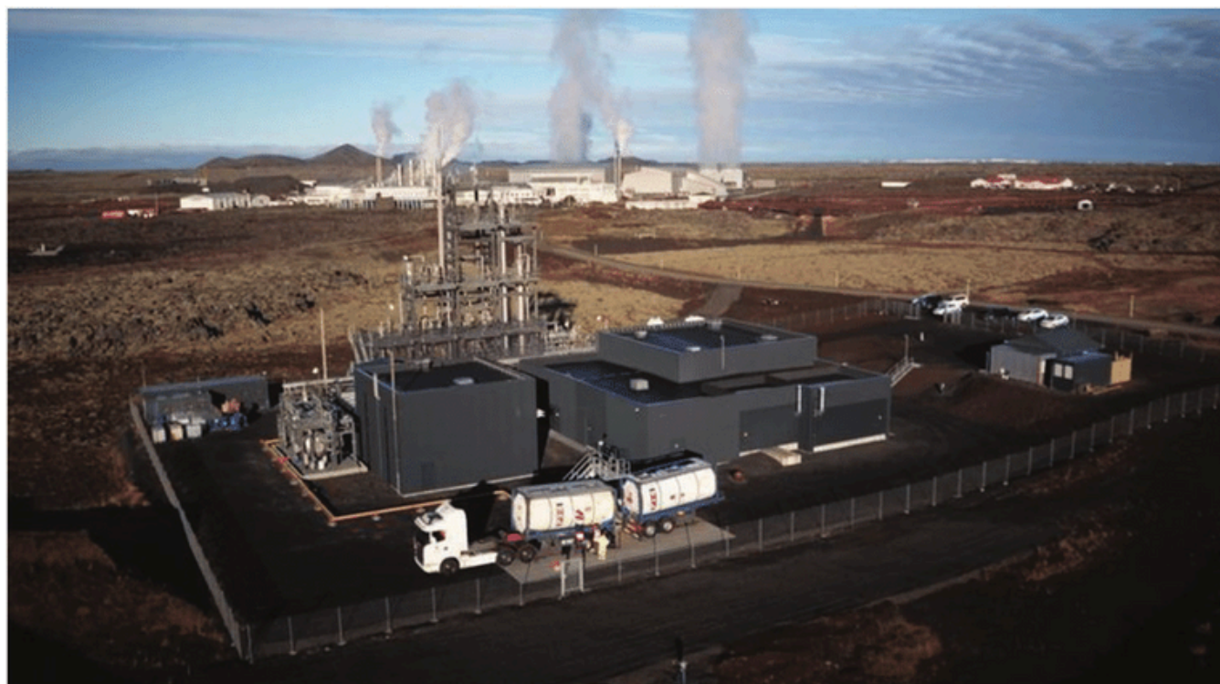
Figure 8. Carbon Recycling International methanol plant
